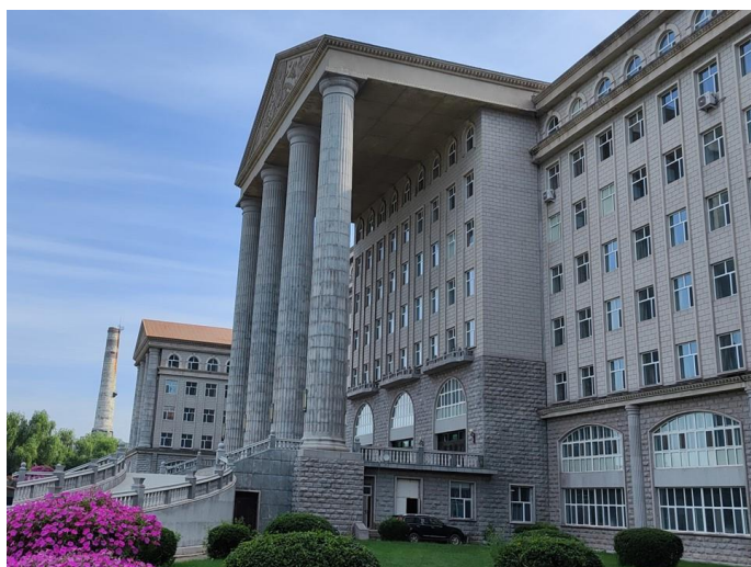
Picture 2.2. Main building of Jilin Agricultural University, the place where ASPT5 was held. The columns of a 7 story building are about 30 m high, and I was informed these granite columns weigh 100 tons each.
